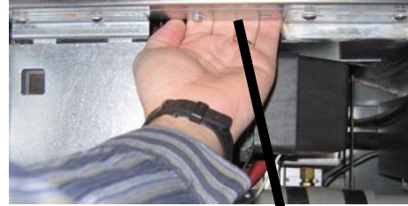
Location of switch on a gas fryer is behind the left control box.
